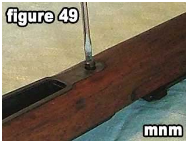
49) Tighten the front guard screw.
